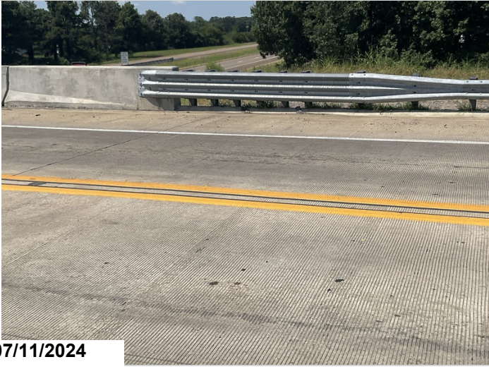
Left side abutment 2 approach guard rail transition.
