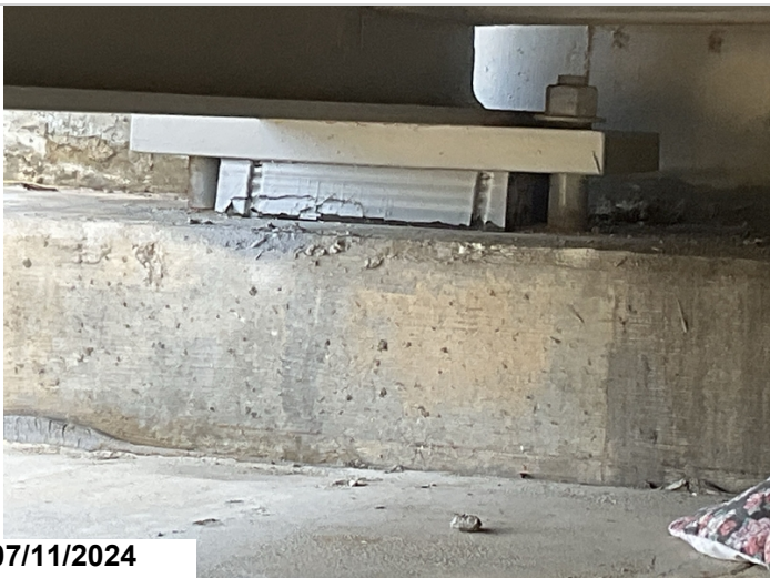
Typical elastomeric bearing.
