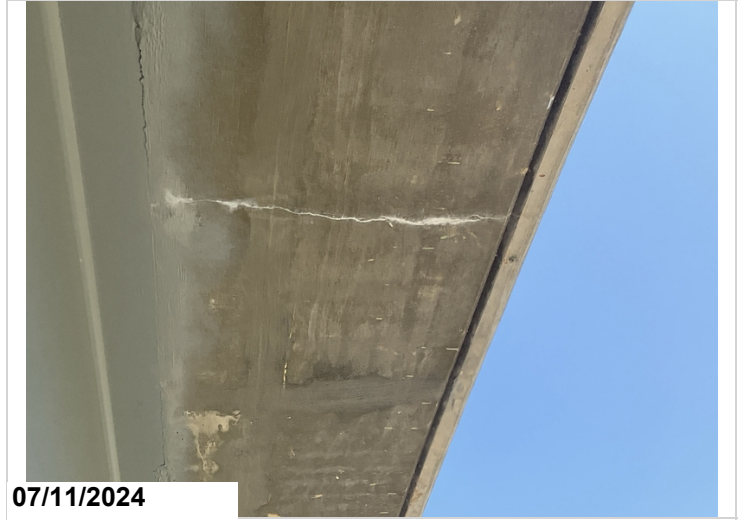
Typical transverse crack right side undersurface.
