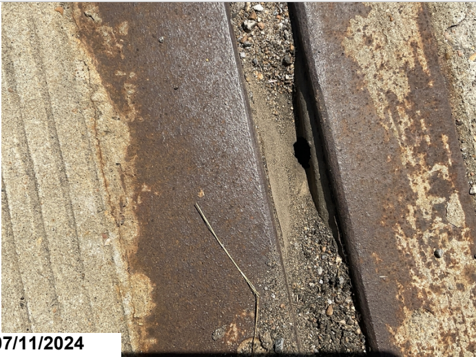
Abutment 2 left side joint seal has small hole.
