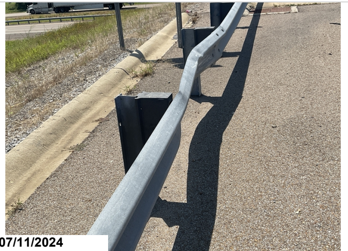
Abutment 2 right side guardrail has collision damage for 6' 12 posts from abutment 2.
