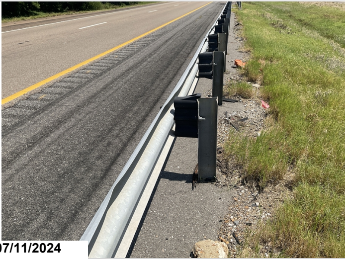
Guard rail has collision damage for 10' 120' east of bridge and 3 guard rail post damaged.
