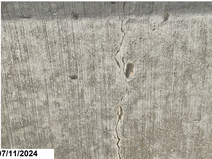
Typical bridge rail crack.
