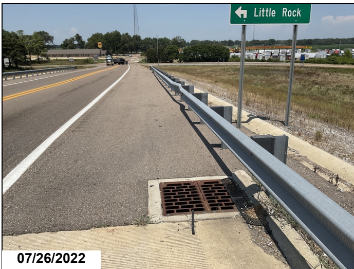
Abutment #2 right approach rail has minor collision damage
