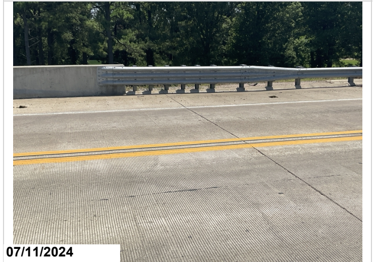
Abutment 1 right side guard rail transition.
