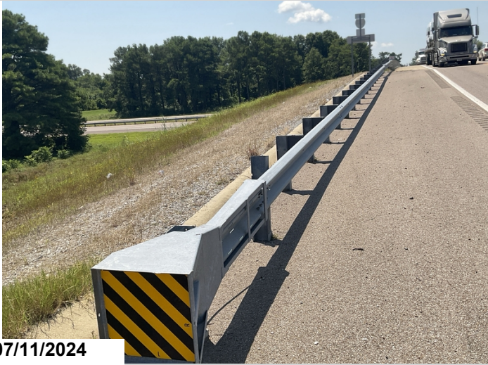
Approach guard rail right side abutment 2.
