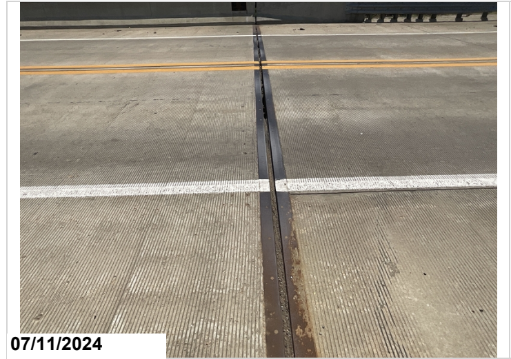
Abutment 1 typical joint.
