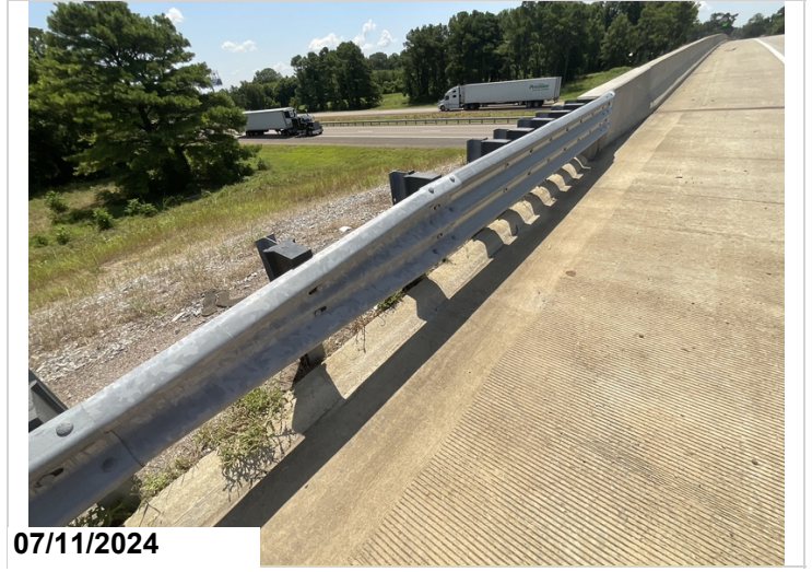
Right side abutment 2 approach guard rail transition.
