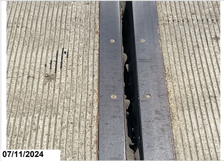
Typical joint seal has fell in for 30'.
