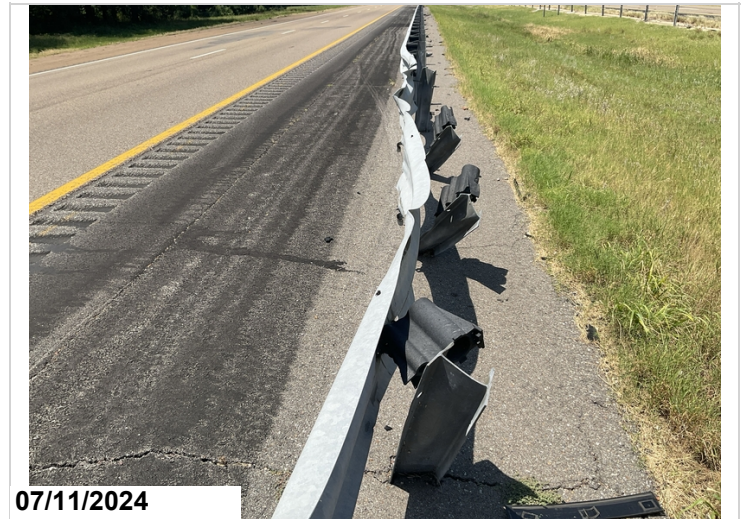
Typical guardrail east bound side 90' west has collision damage for 20' with 4 rail post damaged
