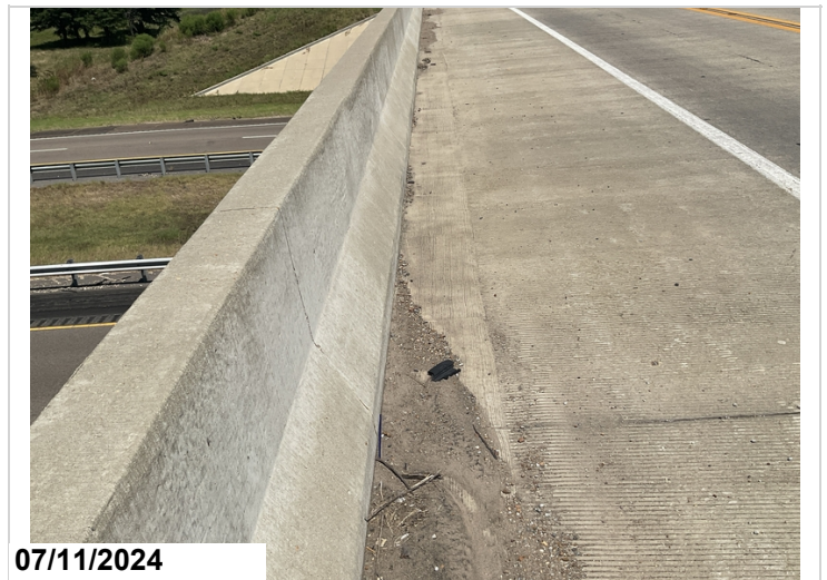
Dirt and debris in gutters.
