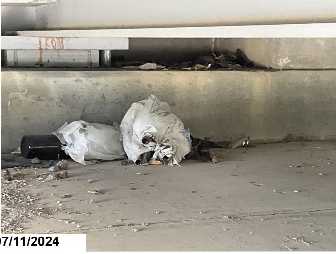
Caps at both abutments have dirt and debris on them
