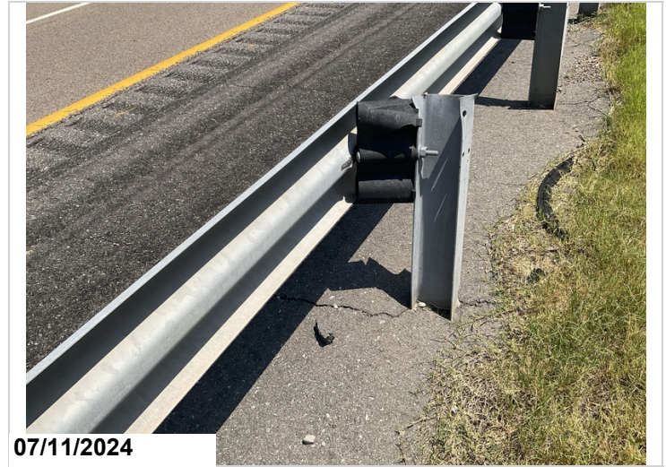
Guard rail posts damaged west bound side.
