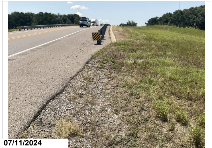
Guard rail end left side abutment 2.
