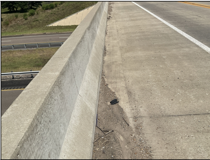
Dirt and debris in gutters.
