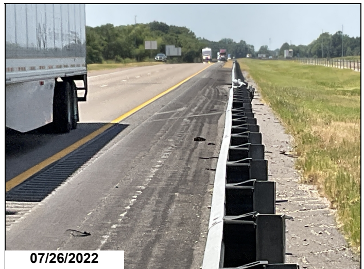
East bound under bridge rail has moderate collision damage.
