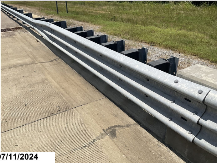
Abutment 1 left side guard rail transition.
